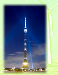
Moscow (Moscow Telecommunications Cop.)
